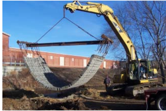
Installing the boat launch
