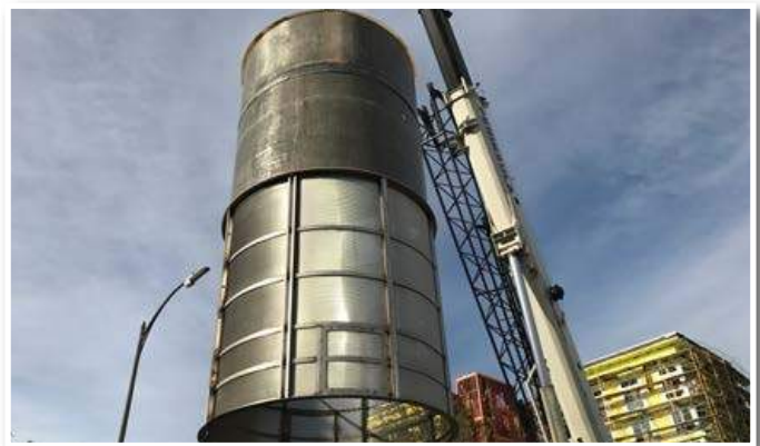
CDS standalone system removes trash and sediment.
