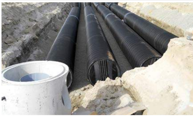
CDS pretreats a rainwater harvesting cistern.
