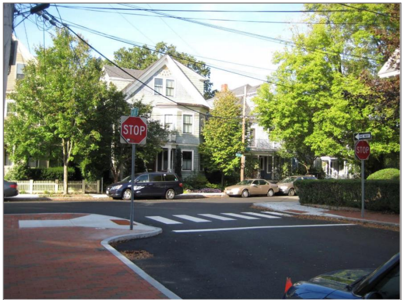
Above: Curb extensions are permanent changes to the street structure that serve to slow traffic and provide additional protection for pedestrians.
